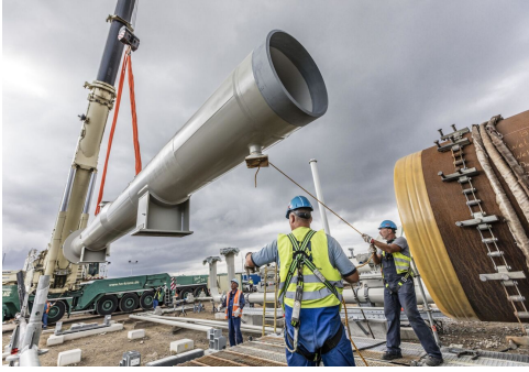
Nord Stream 2 © Photo : Nord Stream 2 / Paul Langrock
